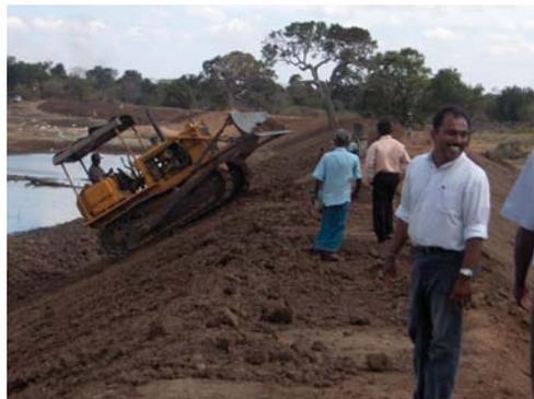
**Figure 3.** Contour lining for soil water conservation bunds.
